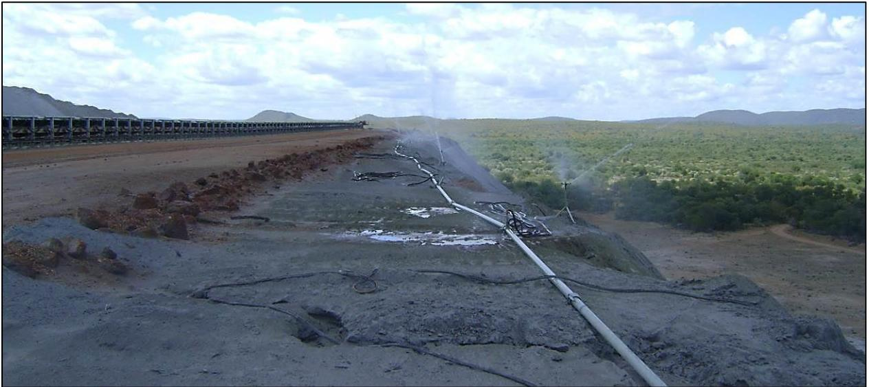
**Figure 8-11: Dust suppression system at Matimba Power Station**
